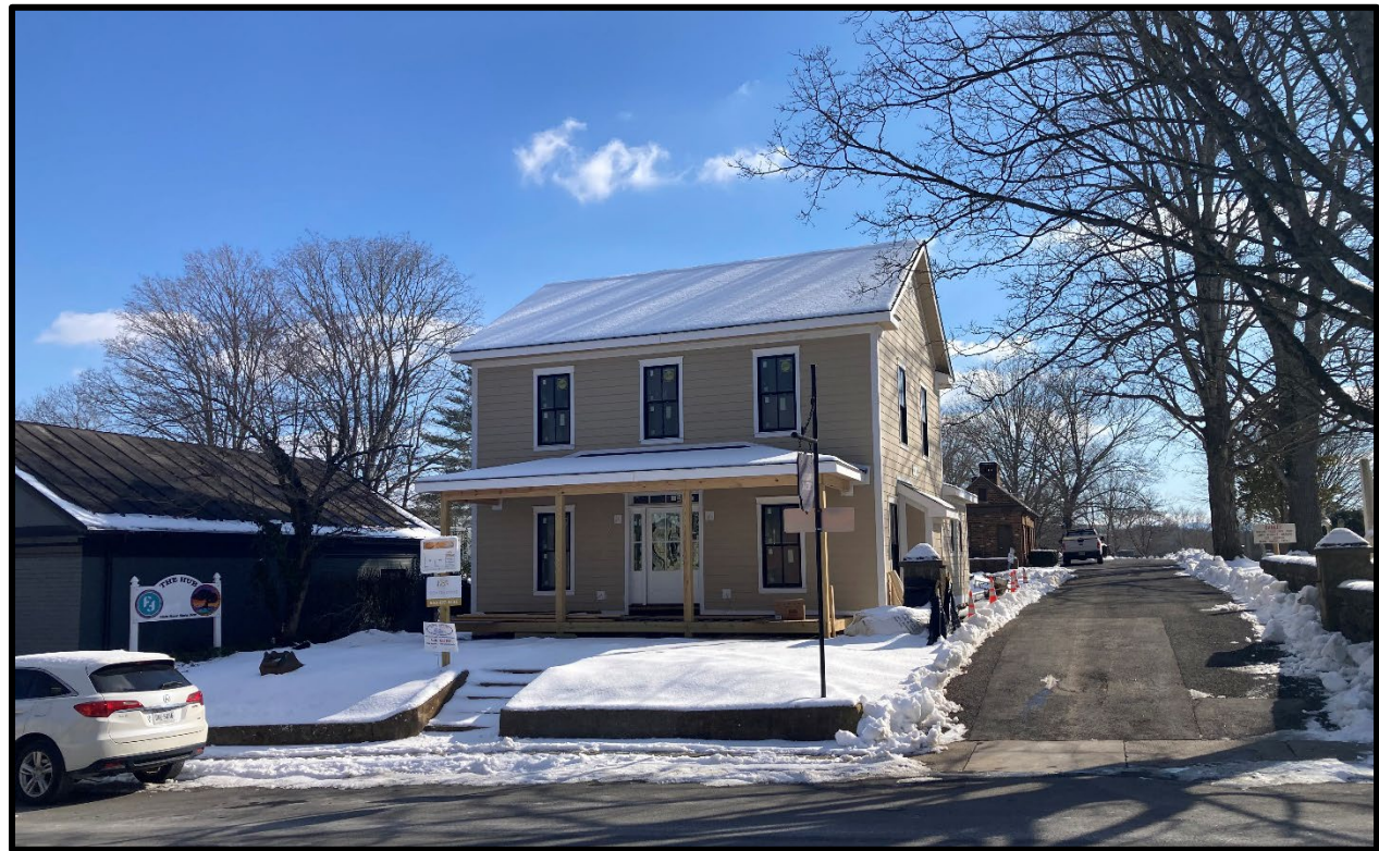
316 South Main Street existing conditions
