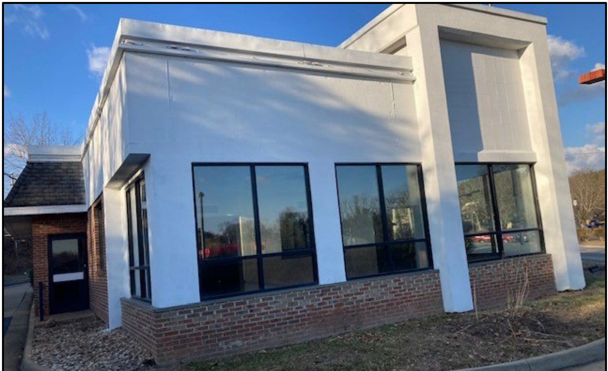
100 Walker Street front elevation
