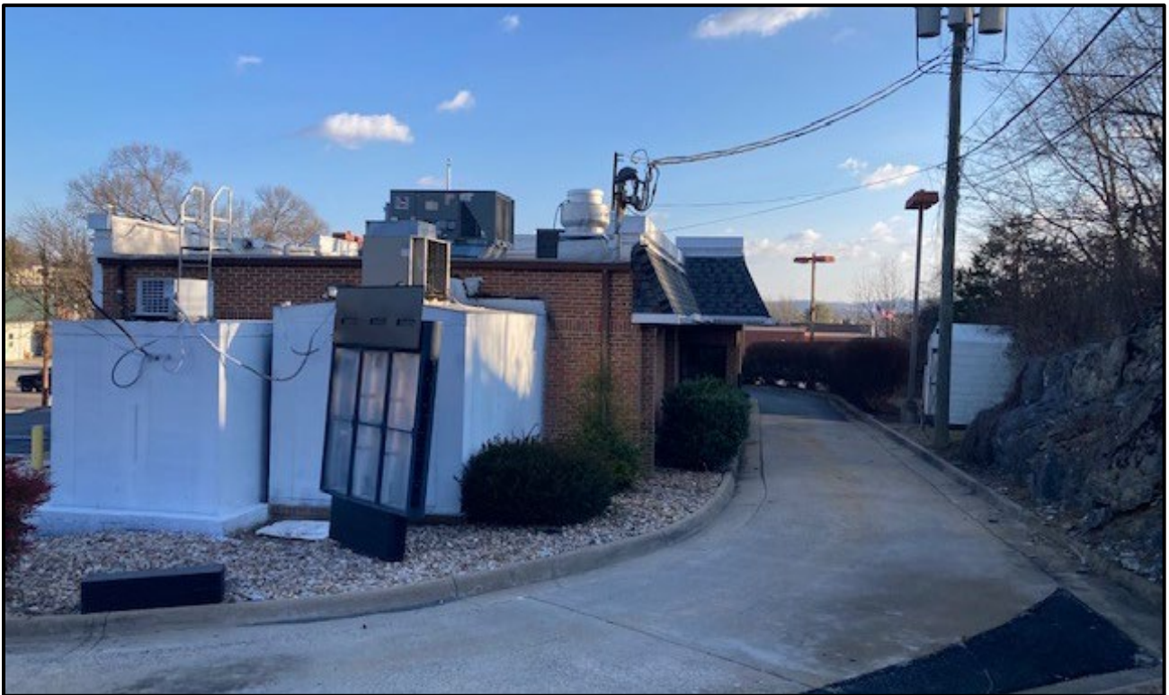
100 Walker Street rear elevation
