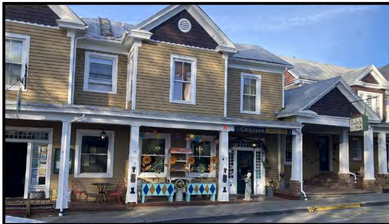
112 W. Washington Street existing conditions (photograph #1)
